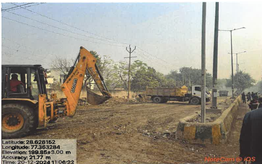
Figure 1: Site Photograph of Mixed Waste on Roads.
